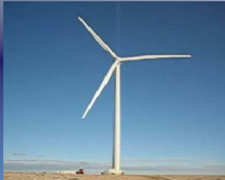
93 Meter Diameter and 2.5MW
